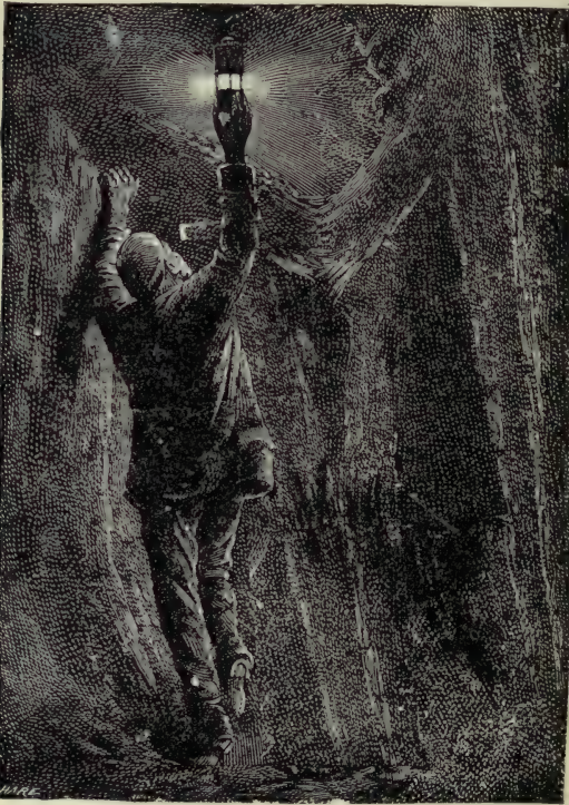
FIG. 65.—Making a Test for Gas
